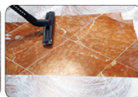
Step 5 When desired finish is achieved, then remove all slurry with wet vac and rinse thoroughly.
