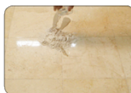
Step 2 Pre-wet a small area with water & add 1-2 cups of Hone 400™ to form a slurry.
