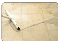
Step 4 Remove some slurry and check on progress of the honed finish.
